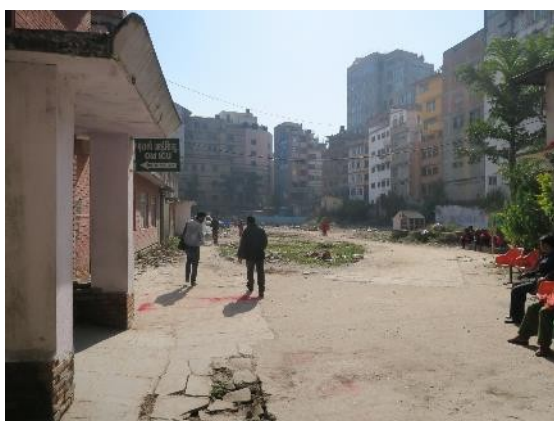
Bir Hospital demolished the severely damaged ward, but securing water source is current problem
