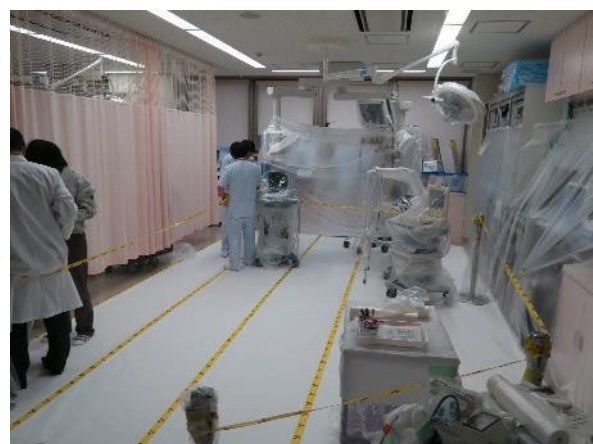
Curing of Radiation Controlled Area (RCA) in ER
